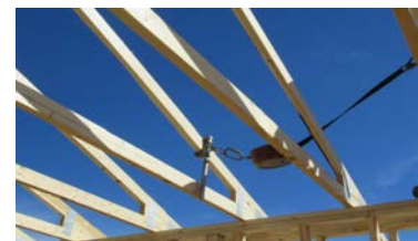
Employee using a beam clamp as an anchor point.
