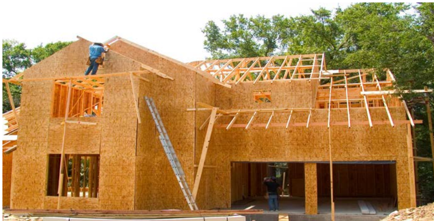
Employee without using fall protection
