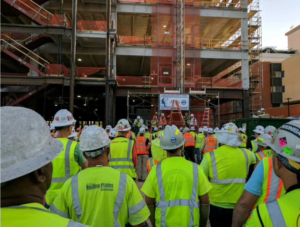
Schultz and Atencio at Sundt and DPR site
