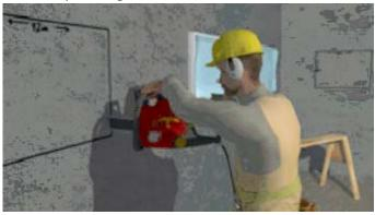
This image, from one of OSHA's animated educational videos on construction hazards, shows a worker using a pneumatically powered saw, rather than one powered by gasoline, to reduce the buildup of carbon monoxide in a confined area.
